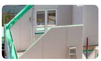
ArmaForm Eco is a suitable core for all kinds of prefabricated structural insulated panels in the building envelope and internal partitions. In addition to its long-term insulation and structural integrity, additional key benefits are its thermo formability into curved shape and its versatility with almost any type of finishing options.
